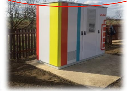
LV: In line voltage control
